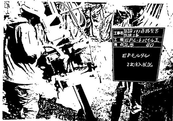
Photo 6.Mortar injection
