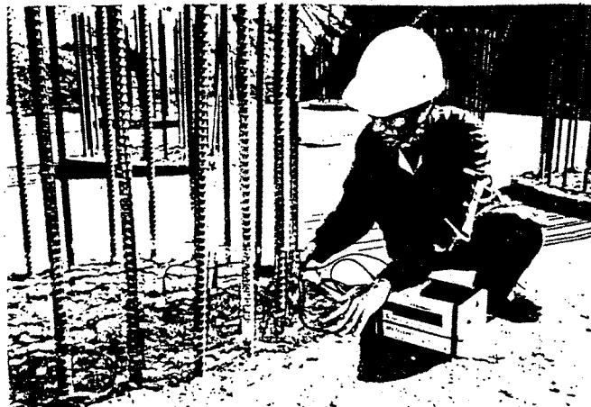
Photo 7. Performance of integrity test
